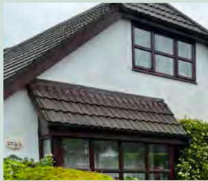
Black tiles on half hip roof
