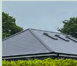
Welsh slate hipped roof with ridges
