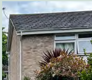
Gabled roof with grey slate
