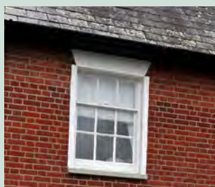
Sash window and rendered lintel
