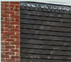
Red brick with clay hung tiles
