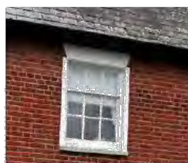
Sash window and rendered lintel
