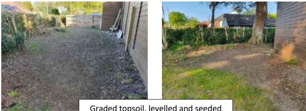
Graded topsoil, levelled and seeded April 2022
